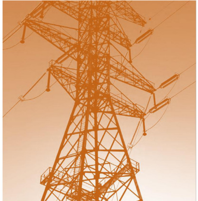
KCP&L and GMO's electric utility system has approximately 3,600 circuit miles of transmission lines
