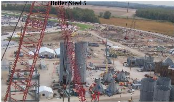
Alstom Fabrication Area 2
