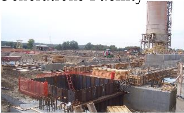
Air Quality Control System West End Foundation Work
